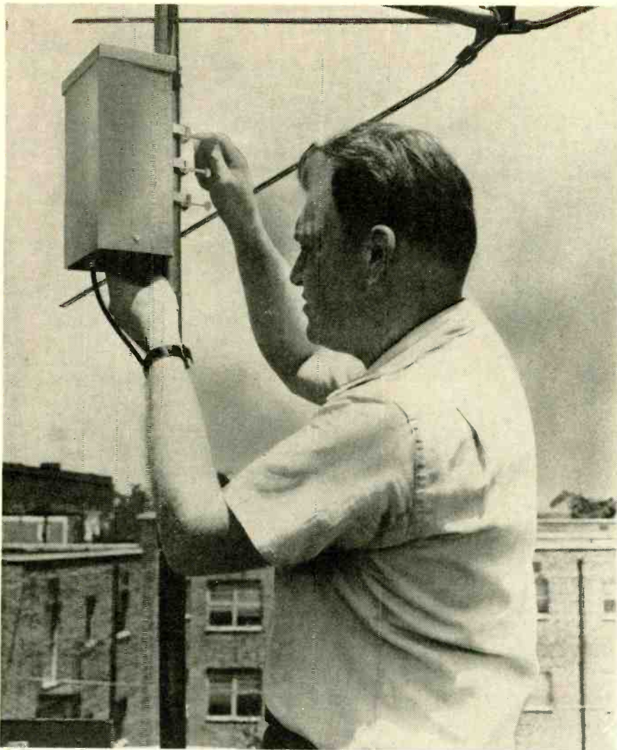
Technician replacing mast-mounted preamplifier
